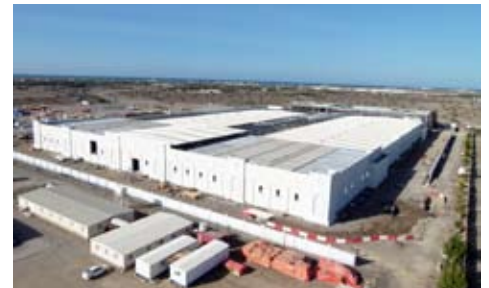
Civil Works for A'Seeb STP
