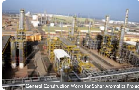
General Construction Works for Sohar Aromatics Project
