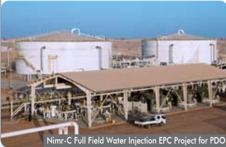
Nimr-C Full Field Water Injection EPC Project for PDO
