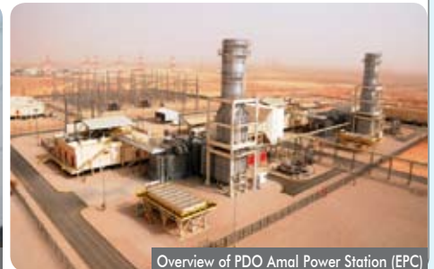
Overview of PDO Amal Power Station (EPC)
