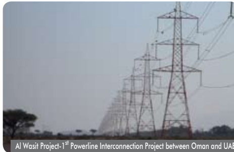
Al Wasil Project-1 st Powerline Interconnection Project between Oman and UAE
