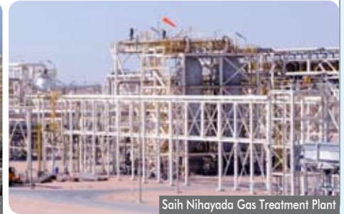
Saih Nihayada Gas Treatment Plant
