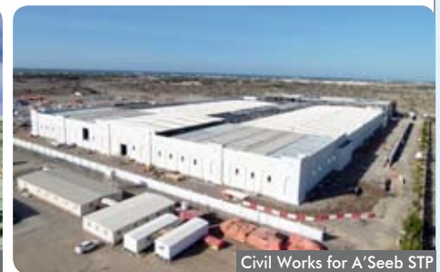
Civil Works for A'Seeb STP
