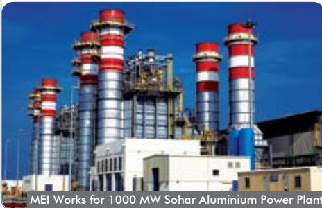
MEI Works for 1000 MW Sohar Aluminium Power Plant
