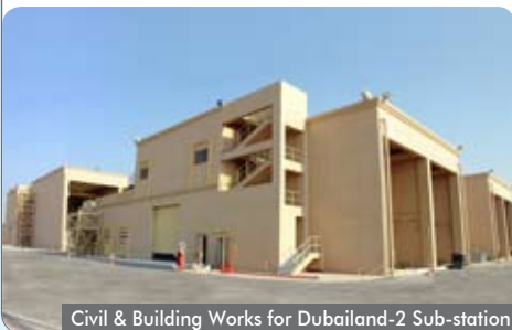
Civil & Building Works for Dubailand-2 Sub-station
